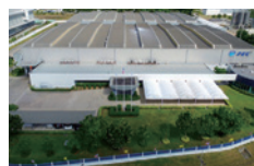
PEC Manufacturing (Thailand) Ltd.
